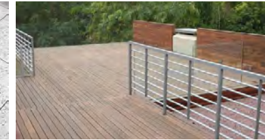
2 Wood Decking on Pedestal System
